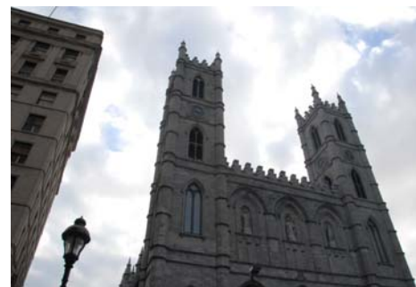
Figure 11 Initial image to be patched
